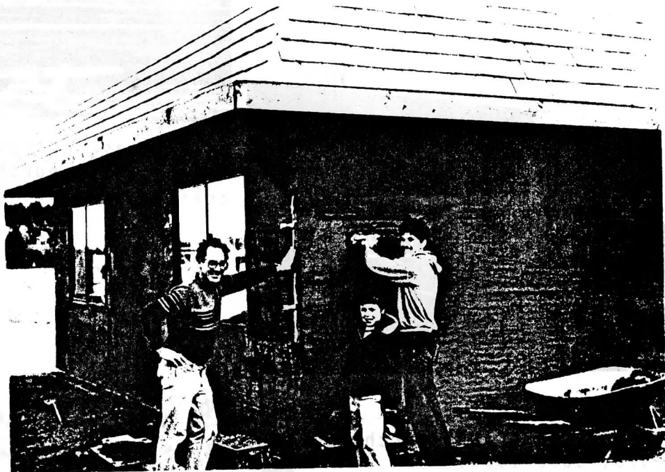
The EXTENSION added on to the downstairs's Club room. Colin Brough, (L); his son Tony; & Frank Benvin apply mud undercoating for stucco. 1989
